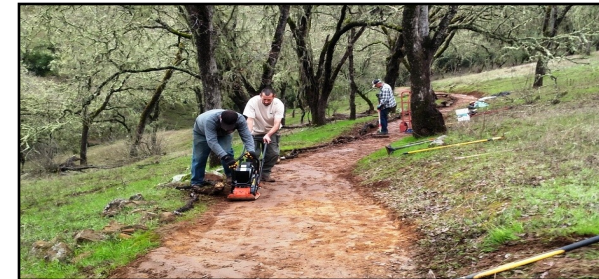
Three Bridges Oak Preserve - trail maintenance
